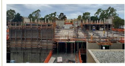
Construction continues with the parking structure. East deck concrete pour for level four is scheduled for 1/3/20 with columns and wall concrete pours following on 1/14/20.
